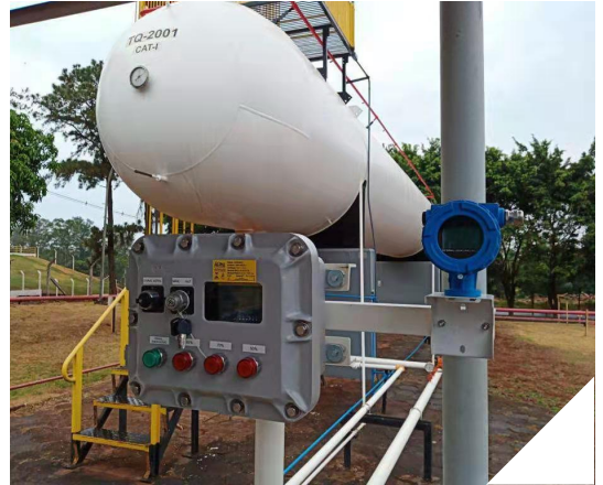
Kryohm level measurement on a bulk storage tank
